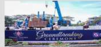
Ground Breaking Grand Taruma Commercial 26 Juni 2021
